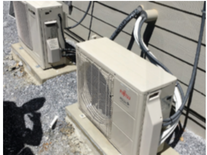
Fujitsu 3/4 ton mini-split heat pump: heating & cooling
