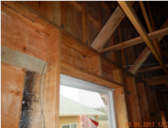
Advanced framing, less wood
