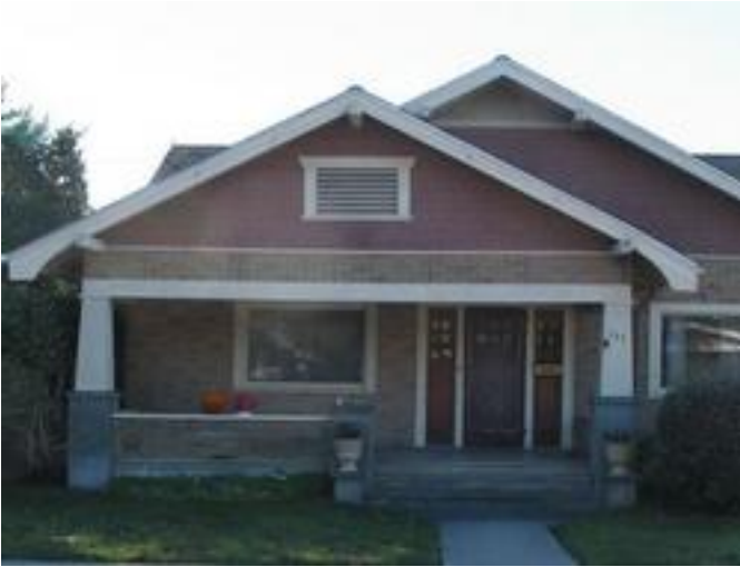
House front Pre
